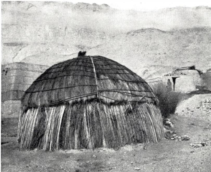
Fig. 5. 'Chapar' completely covered with straw from the Hazāra between Dōshi and Pul-i-Khomri. The frame consists of curved sticks and there is no central pole. This type is also found with mats and felt cover. (Phot. by Peter Rasmussen, November 1953).
